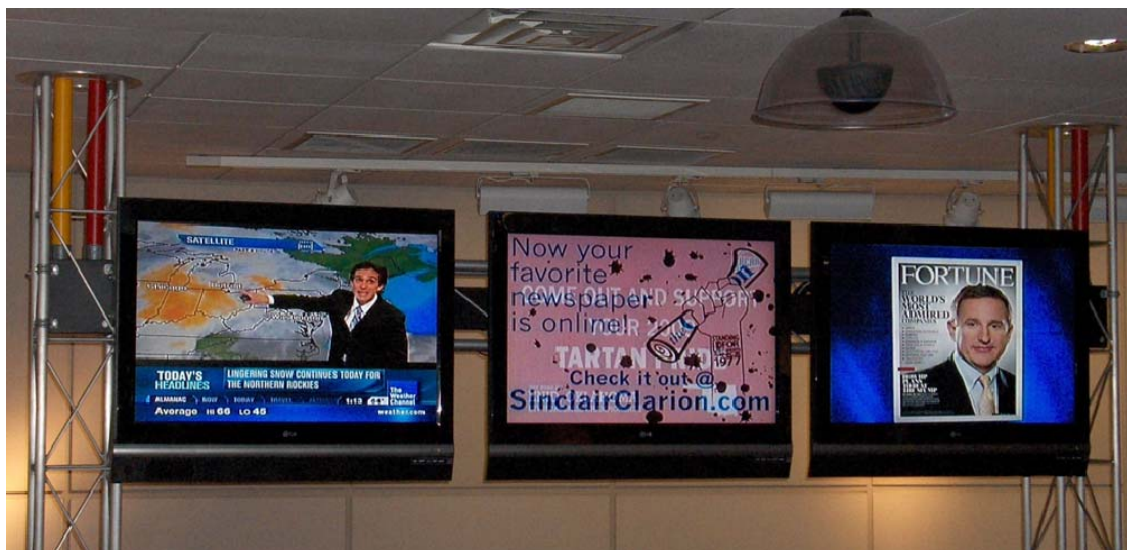
Figure 3-23. The campus cable TV system displays multiple types of video in Building 14.
