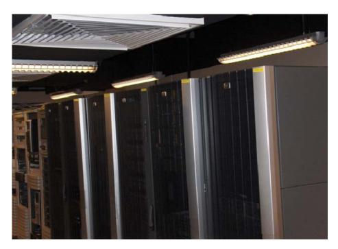
Figure 3-27. Server Room with vents for improved airflow and without ceiling tiles.
