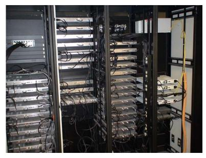
Figure 3-34. Racks of equipment in the campus' cable television head-end.
