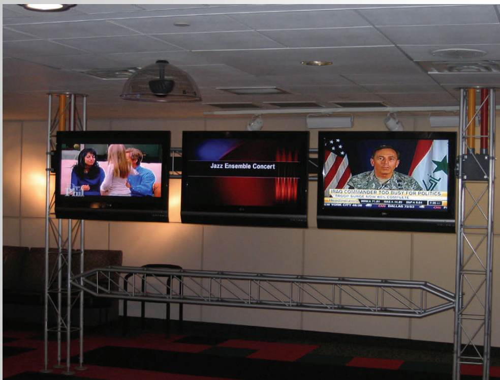
Figure 3-32. The replacement for the video wall displays CastNet and campus cable system content.
