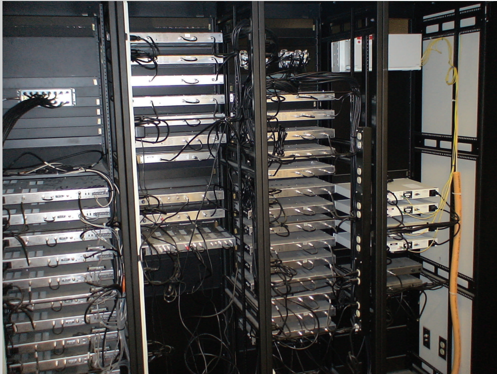
Figure 4-18. Racks of equipment in the campus' cable television head-end.
