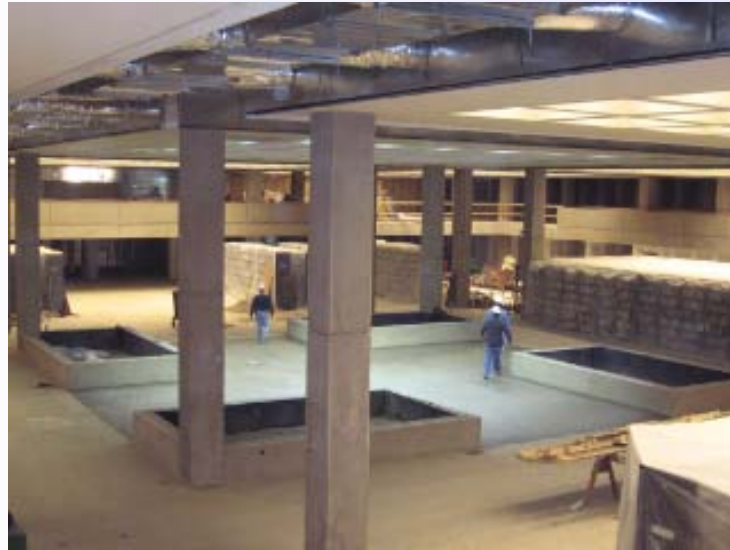
Figure 3-4. Library Renovation In-Process.
