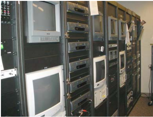
Figure 3-46. Cable head end (left) and a Building 12 conference room (right).
