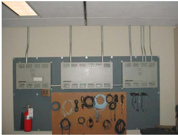
Figure 4-25. Building 12 lighting (left) and sound (right) control equipment.
